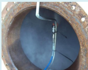
Fogging of Ox-Pro™ 137 into void spaces for asset corrosion protection
